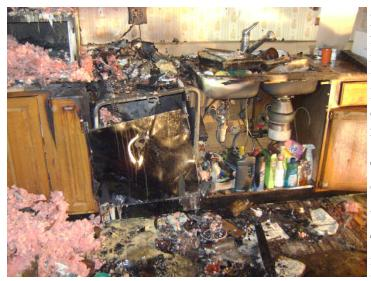
May 6 - An electrical fault ignited a dishwasher. The fire extended to the upper wall cabinets. The fire melted a plastic water line that supplied the dishwasher, extinguishing most of the fire. Despite the limited fire spread, heat and smoke damage to the condominium unit was extensive. Workers were still repairing the damage in mid-September.
